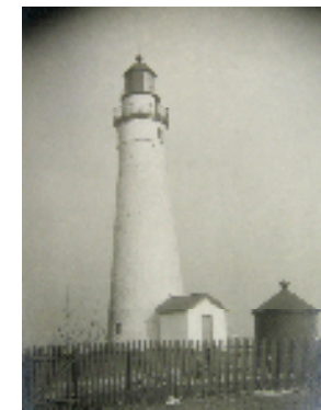
Fort Gratiot Lights Station Tower circa 1913
